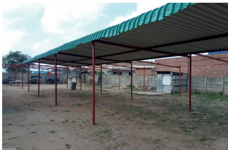
New market under construction, Mbizo 4 Shopping Centre. E Nyoni, 2023
