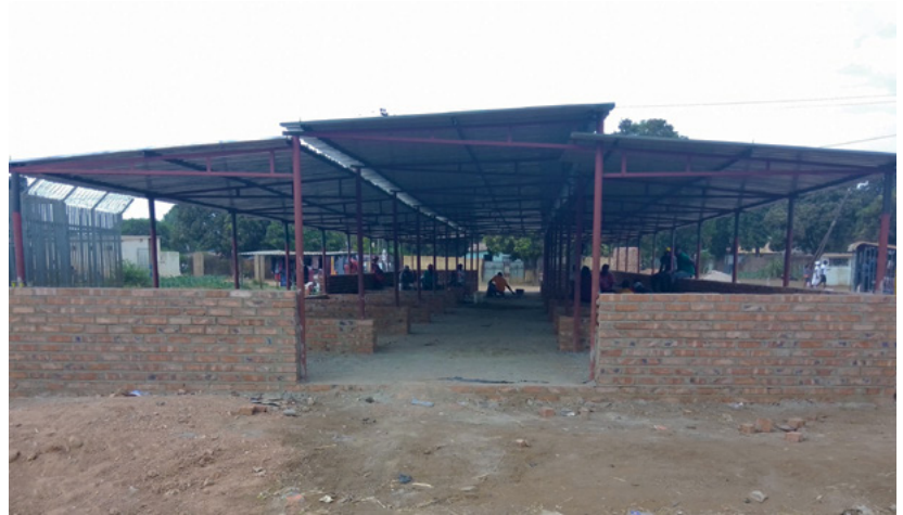
WHH funded Pfulajena market under construction in 2022. D. Murambadoro 2022
