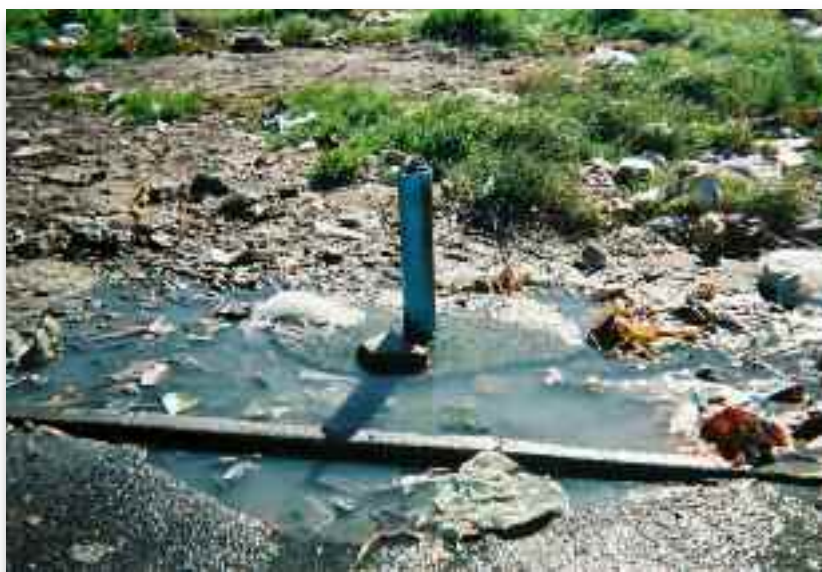
Poorly maintained water services, South Africa
