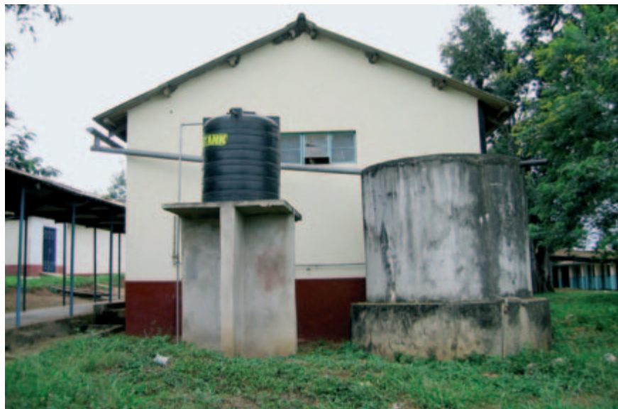
Two containers collecting both rain and municipal water at a district hospital (Tanzania)
